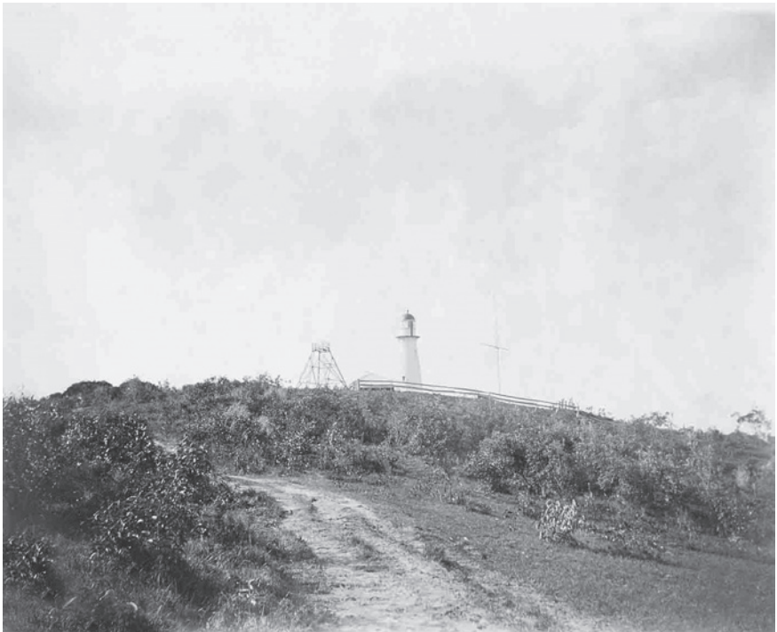
Early photograph of Bulcock’s watch tower, lighthouse and cottage.
